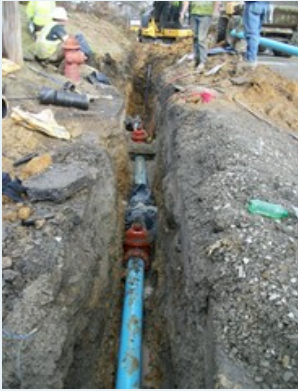
(New Distribution Pipes)
