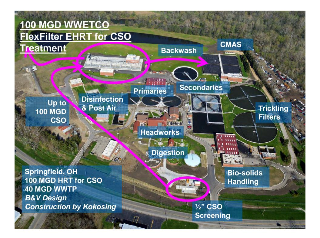
High-rate / high-performance / small footprint No chemicals required to remove solids Operating power less than \$5 per million gallons treating CSO Operating power less than \$1 per million gallons when polishing
