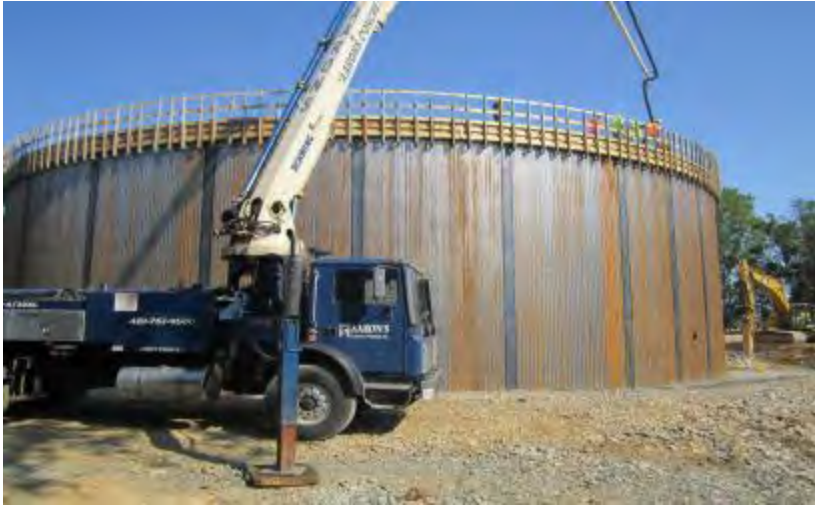
3 MG of Storage DN Tanks Concrete AWWA D110 Tank
