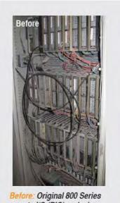
Petore: Original 800 Series remote I/O (RIO) racks in dryer area main control enclosure.
